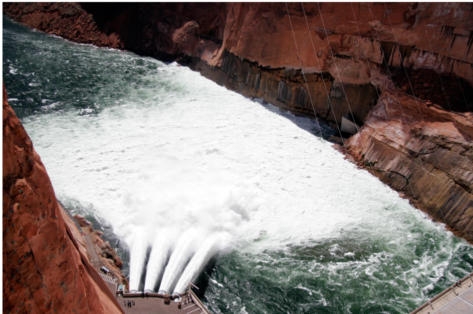
Figure 40. Views from below Glen Canyon Dam, looking upstream (top) and from the top of Glen Canyon Dam of jet tubes during 2008 HFE (bottom). Bottom Photo: T. Ross Reeve via USBR.
