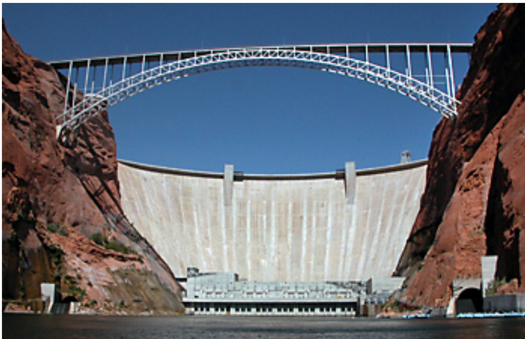
Figure 22. Photograph of Glen Canyon Dam and Power Plant (USBR 2009).
