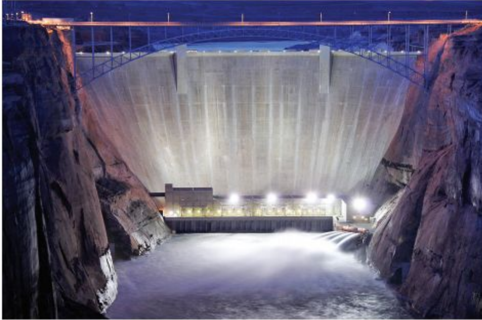
Glen Canyon Dam releases high flows of Colorado River water on the night of March 6, 2008. A high-flow experiment was undertaken to determine if water releases designed to mimic natural seasonal flooding could be used to improve a wide range of downstream resources in Glen Canyon National Recreation Area and Grand Canyon National Park. (Photograph courtesy of T. Ross Reeve, Bureau of Reclamation.)
